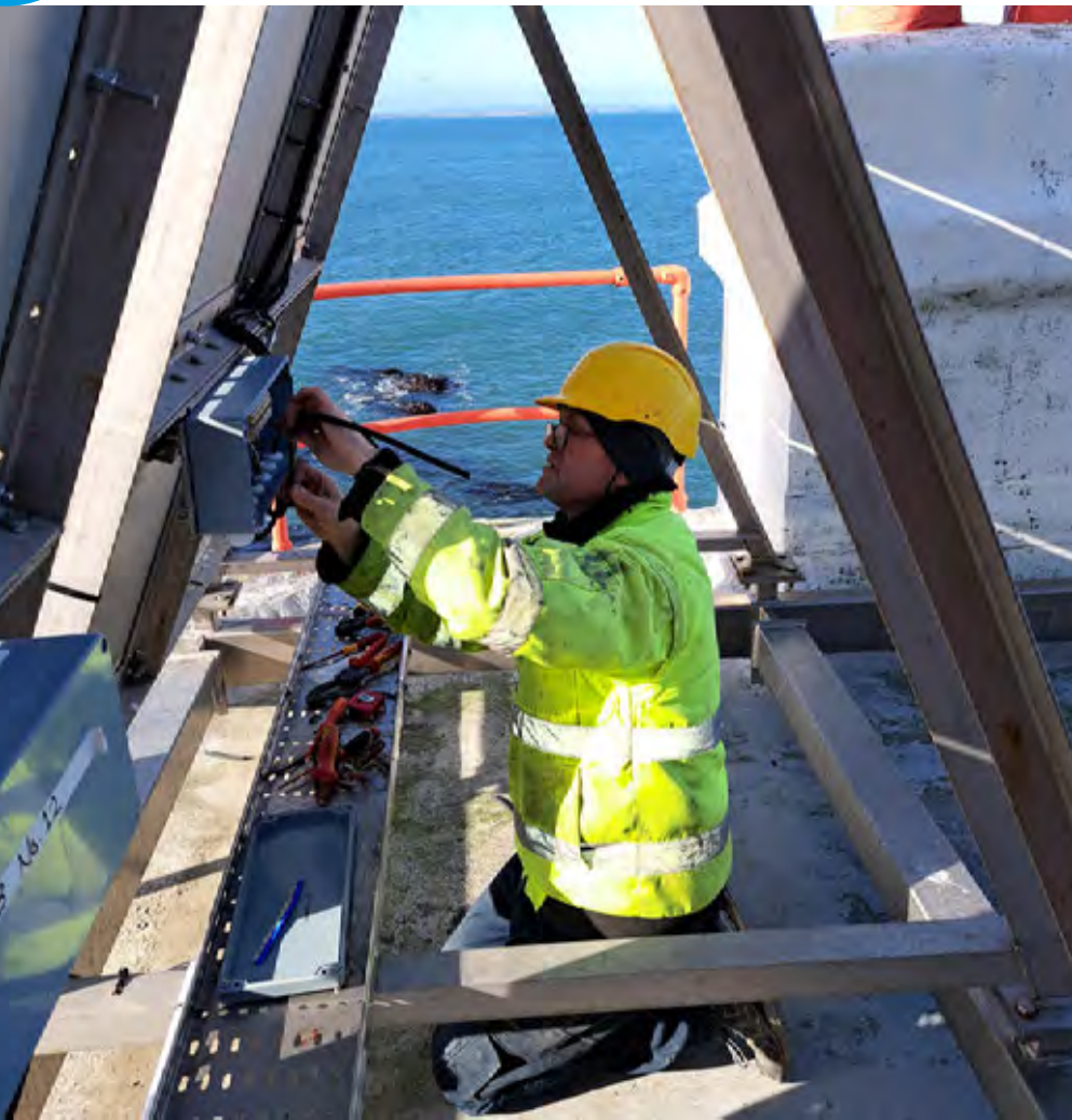
Working taking place to connect the solar panels on one of the three solar arrays at the Tuskar Rock Lighthouse during the significant project to solarise the lighthouse.
